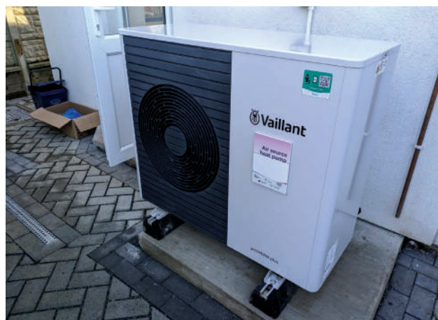
Figure 47. Image of a typical air source heat pump.
