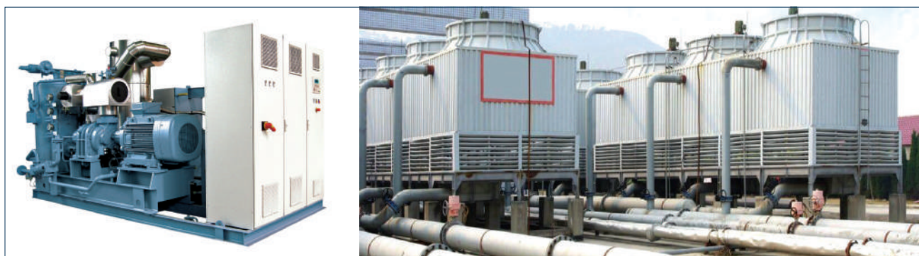
Figure 40. Example of water-cooled chiller (left) and Cooling Tower in a Water-cooled chiller system (right)
