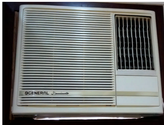
Figure 35. Example of window air-conditioner.
