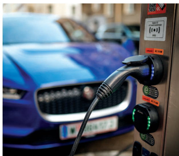
Figure 15. Example of EV Car Charging Ports in Public Car Parks
