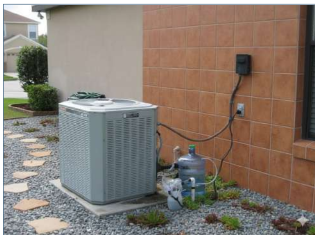
Figure 56. Air-conditioning outdoor unit with condensate water collected in a plastic receptacle.
