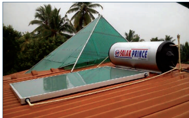
Figure 46. A typical solar hot water system – collector plate with the cylindrical hot water tank.
