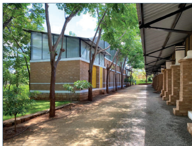
Figure 60. Construction with Stabilised Soil Blocks.
